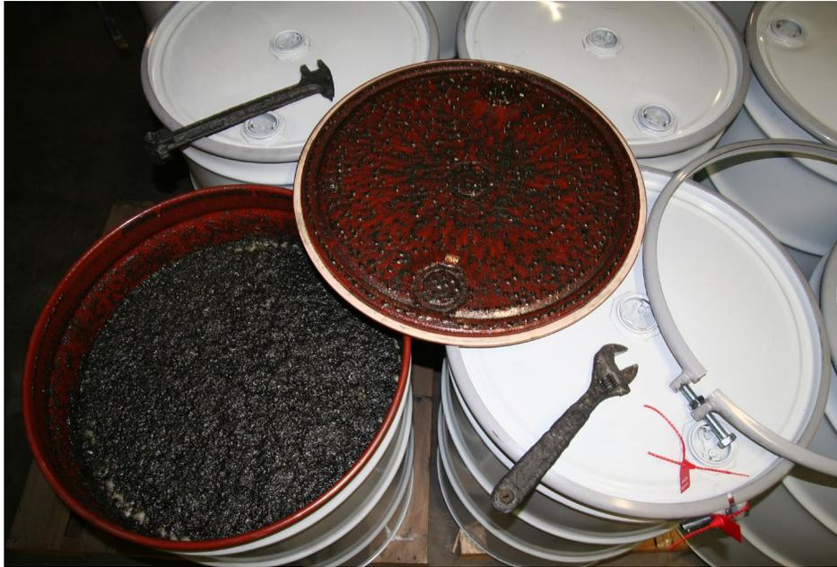
Remove ring and lid. Set aside and keep clean. Replace lid back on drum after mixing.
